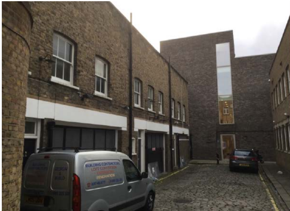
Application site to the left, recently completed student halls development at end of street.
